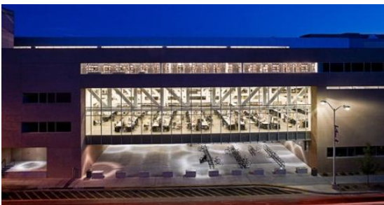
Figure 6. South View at Night (Courtesy: Kirk Gittings, Photographer)
